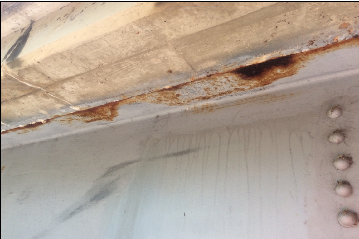
BEAMS RUSTING VARIOUS LOCATIONS
