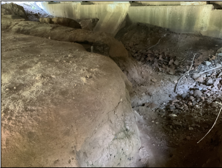
Erosion starting at end of bridge
