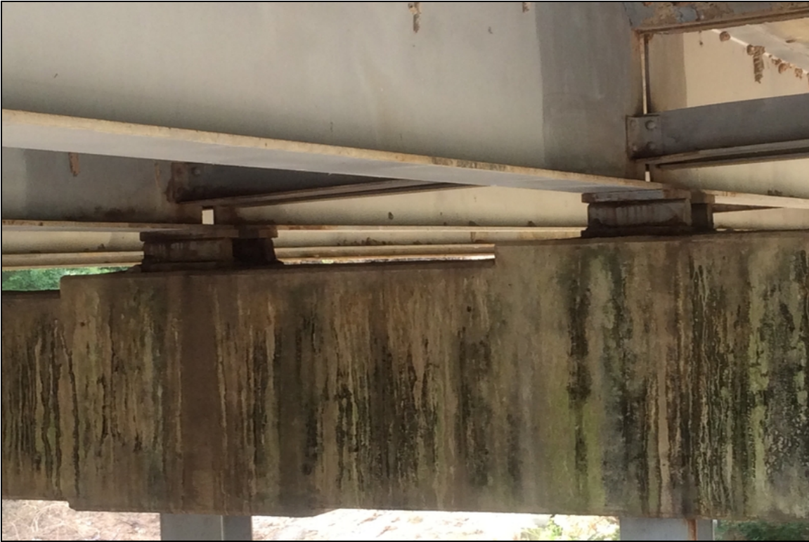
ALL BEARINGS ARE RUSTING ENTIRE BRIDGE H-PILE AND BEAMS ALSO RUSTING VARIOUS LOCATIONS.
